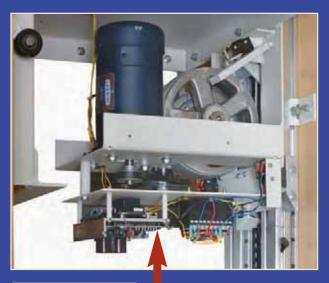
Electric motor, cable-drum drive system and limit switches are pre-installed under car.
